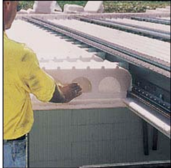
patented floor / ceiling system with light weight beams
