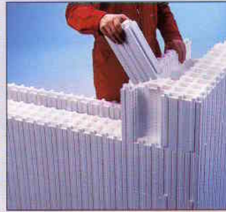
3. Openings at wall ends, corners and T-junctions are closed with end pieces.
