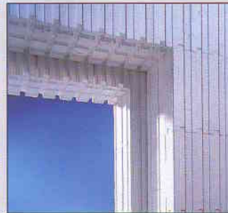
7. The insulation detail at windows reduces heat loss through the window frame.
