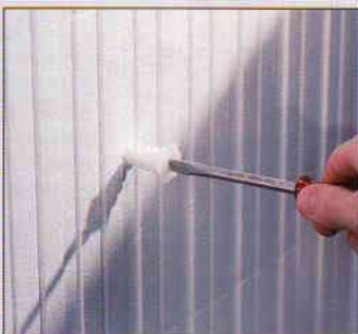
17. Lightweight fixings with the Isodübel plug into insulation foam; heavyweight fixings into concrete.
