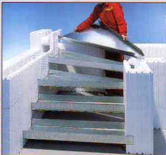
9. Stairs: isorast stair trays are inset into the wall and concreted when the wall is filled.
